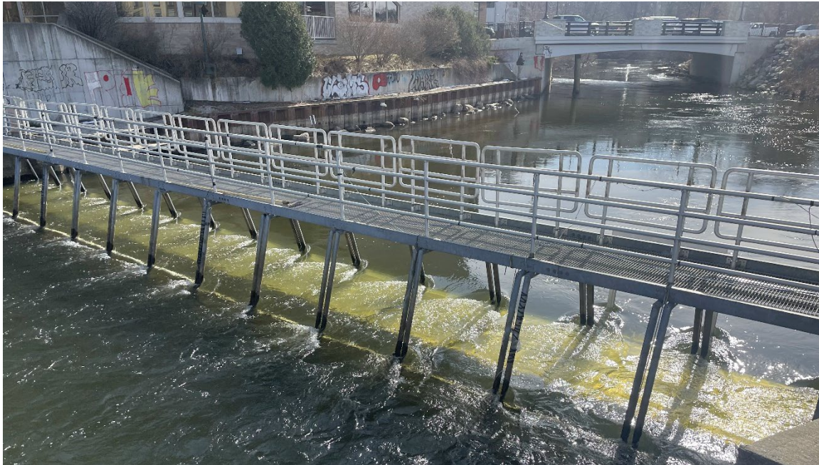
Figure 2. Horizontal submerged screen weir (HSSW) installed at the MI DNR Traverse City Salmon Weir on 18 March 2025. The HSSW is designed to capture a portion of sea lamprey migrating along the bottom of the river while allowing other fish to swim past. If successful, the HSSW could help researchers assess sorting technologies at FishPass.
