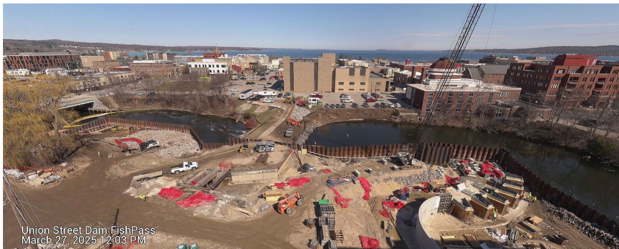
Figure 1. Image capture from the FishPass time-lapse camera: March 27, 2025 showing the initial concrete pours for the arc-labyrinth weir (right side of image) and partial demolition of the existing dam (left side of image).
